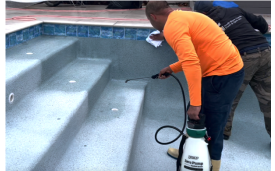
MicroGlass Application on New Residential Pebble Finish
